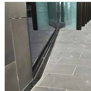
ABOVE: ACO KlassikDrain KS200 with Wedgewire Heelsafe anti-slip 5 star grate at Chelsea Bay.
