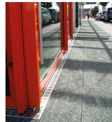
RIGHT: ACO Cantilever ThresholdDrain with Ductile Iron Heelsafe anti-slip grate at Christchurch Justice & Emergency Services Precinct – Te Omeka.
