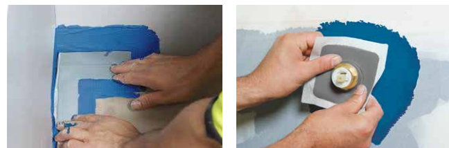
ABOVE: Application of the easy-to-use Gripset Elastoproof bond breaker system.
